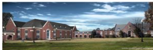
Additions and Renovations to Ramona Woods Hall Jacksonville State University Dr. William A. Mathan, President
